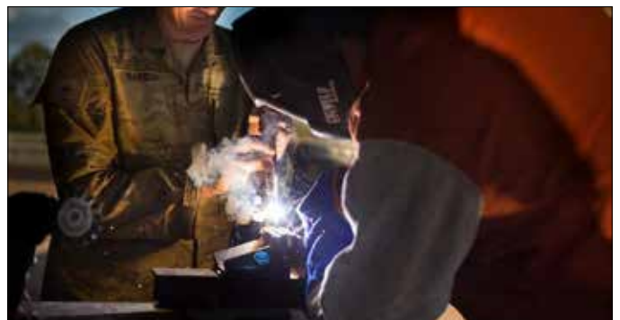
The welder still at work
