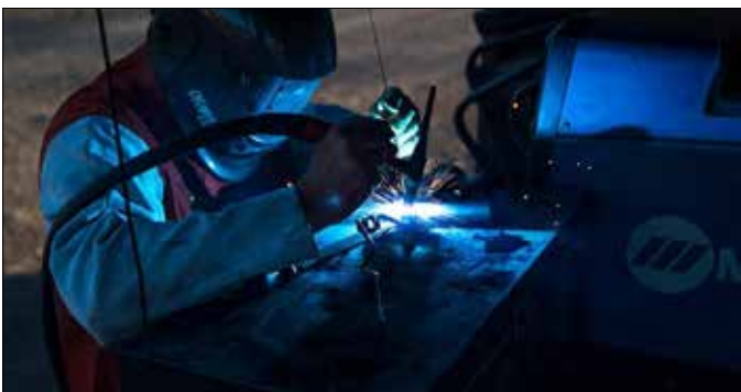
The welder at work
