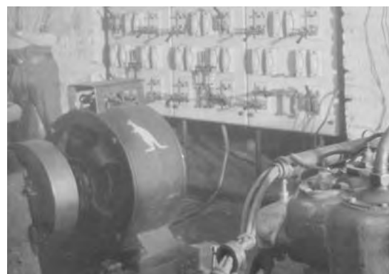
Switchboard of the engine room in an old cellar in the communications trenches at the side of La Basse Canal, Givenchy 1918 (SPR J.A. Lockrey).
